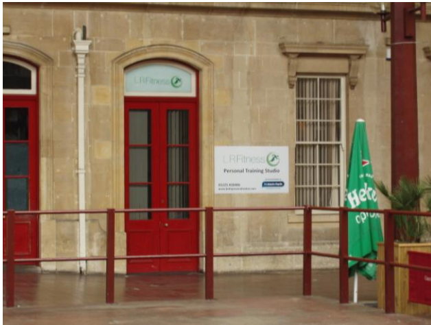
LR Fitness installed January 2014
