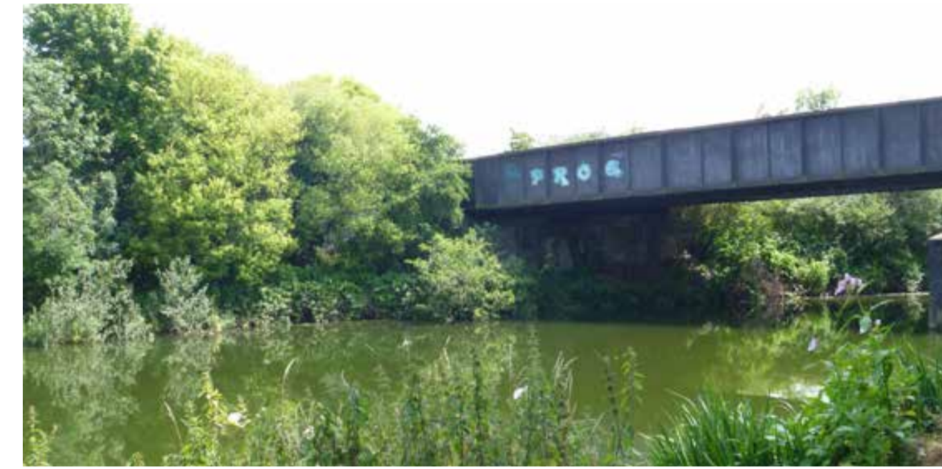
Existing disused bridge over river. Trees obscure site edge to the right.
