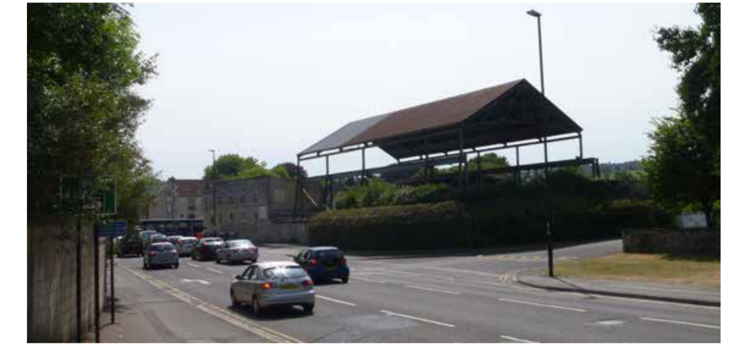
Windsor Bridge road looking south. Existing open roofed structure currently occupies site to right.
