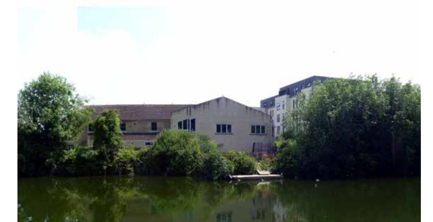
Looking south. Existing church hall and Unite student scheme to right.
