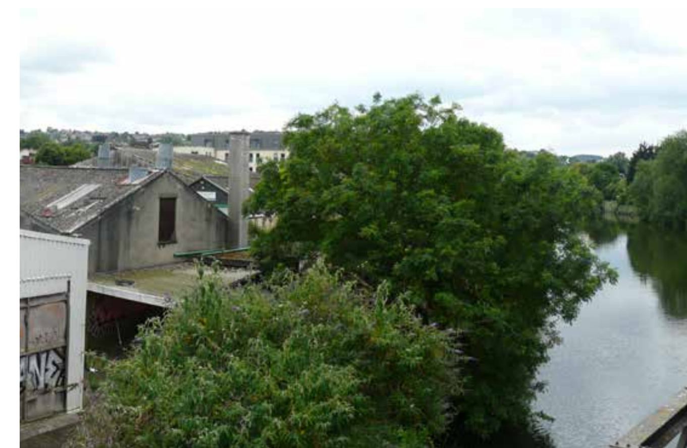
Elevated view from former rail bridge. Site to left bordered by trees.
