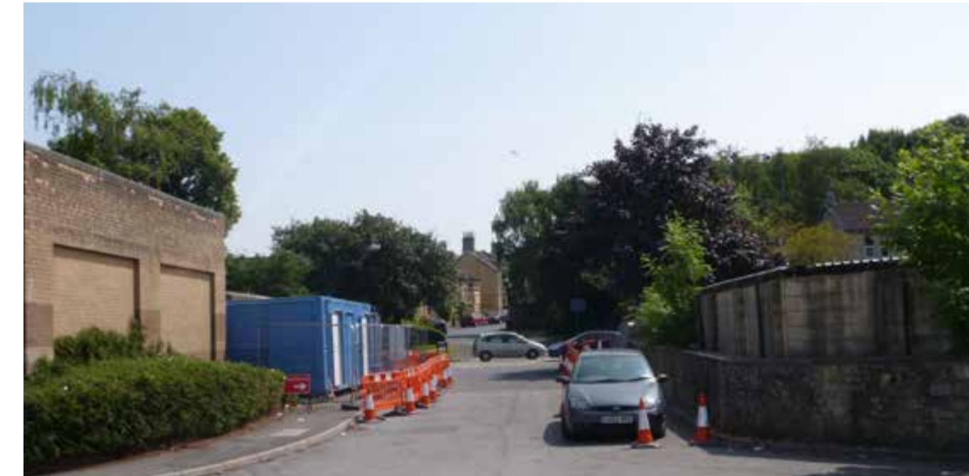
Looking south toward site entrance and Bellotts road junction with Lower Bristol road.
