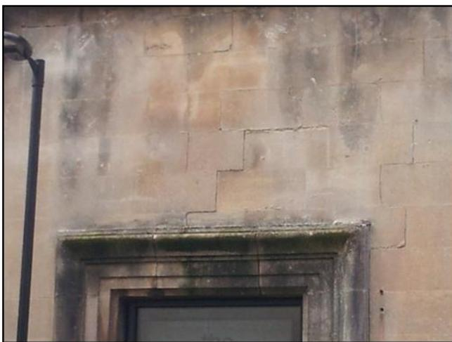
With respect to the offset lettering (and the bracket for the projecting sign, we have concerns at the damage that will be caused to the stonework. As the picture to the left illustrates, cracks are appearing in the stonework where the signage is proposed, which is of concern. We therefore do not consider it wise to drill into the stonework in case this causes further damage. We also note that other cracks are also appearing in the façade of the listed building.
