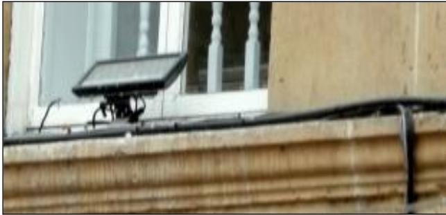
On the station building, the desire to replace anti-roost bird wire with spikes suggests it is either an unnecessary luxury or else there is a trades description problem with the wire currently installed. Closer inspection suggests that the wire would have worked if unauthorised additions had not created perches above the wire.
