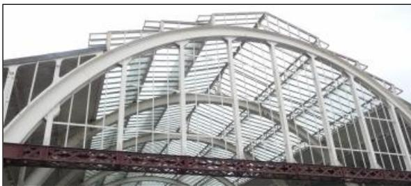
The end of the train shed was originally glazed (the glass was lost during the war and not replaced). If anything has to be used to block off this end section it should be glass, which will maximise the light available in the roofed area while posing as a barrier to birds.
